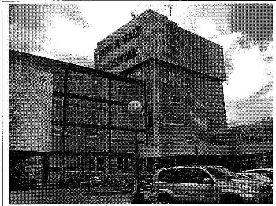
Southern elevation including tower windows
