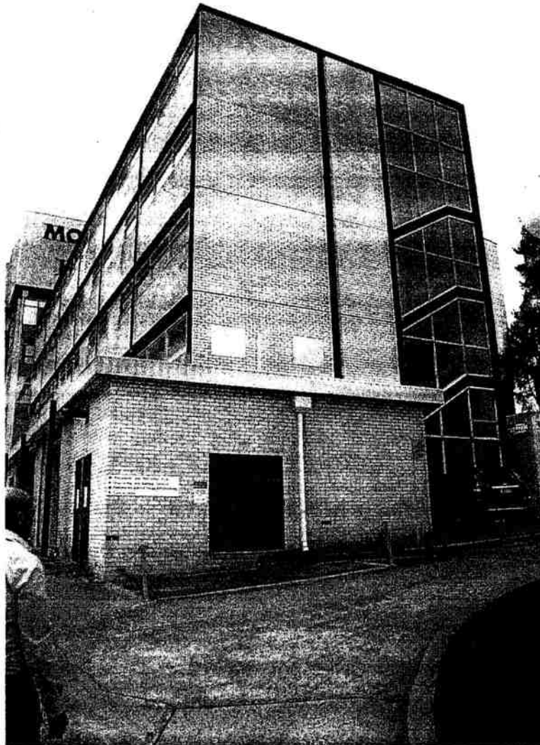
Image 5 - (area 2.2) Wall connecting North-West and Southern Elevation
