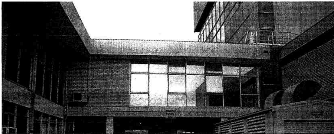
Image 10 - Ambulance entry area of the hospital.
