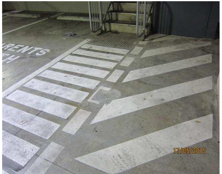
Southern most Walkway, Lower Ground Level.
