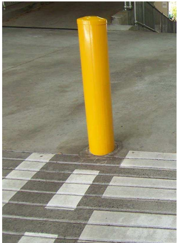
Bungan Lane Car Park – Photo shows the bollards mounted in the core holes
